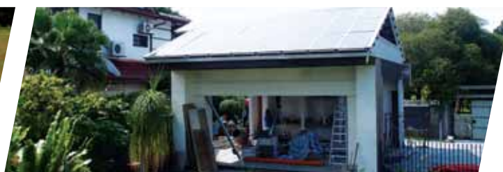
RESIDENTIAL, KELANA JAYA, SELANGOR System Size 11.76 kWp
