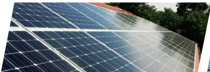
RESIDENTIAL, BUKIT JALIL, KUALA LUMPUR System Size 6.5 kWp
